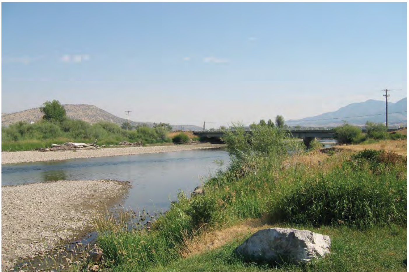
Cardwell Bridge FAS - Jefferson River near Whitehall
